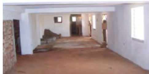
Progress of Sunday School Addition
